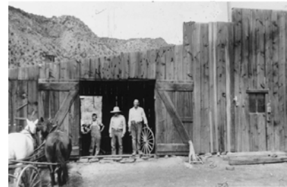
1920s Blacksmith shop
